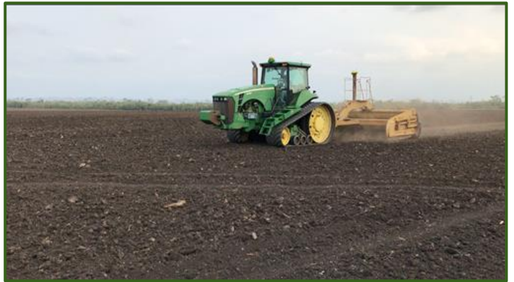
Contour leveling underway
