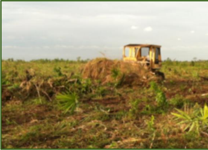
Heavy Tractor pushing debris into “windrows” piles
