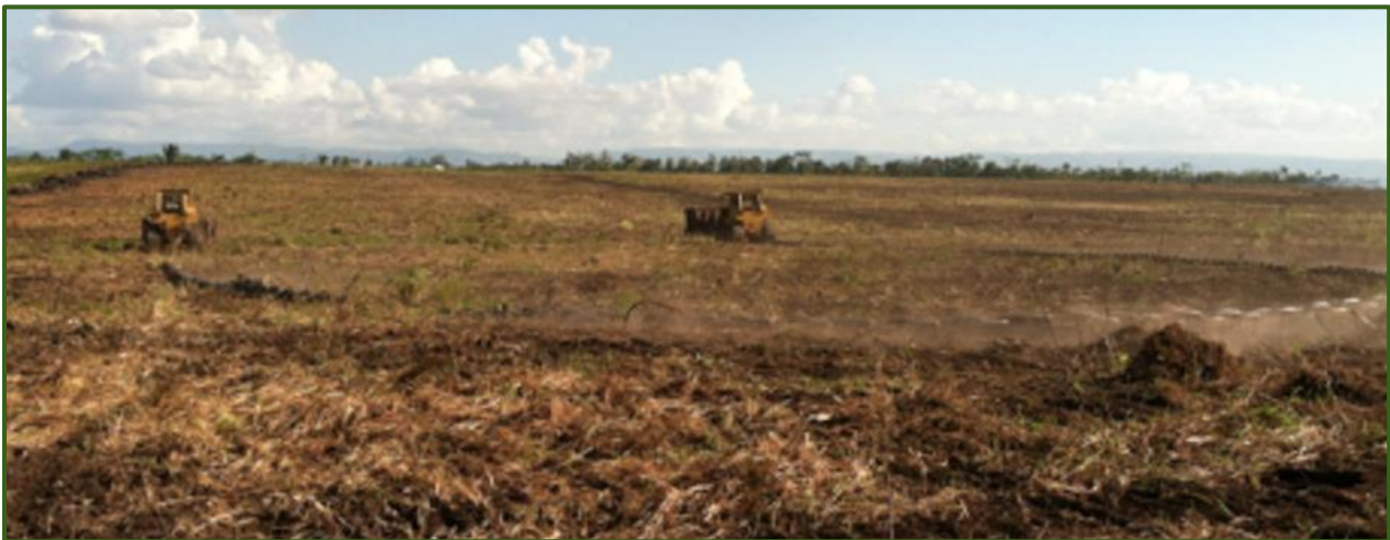
Heavy Bulldozers pulling chain through fields to extract stumps and debris
