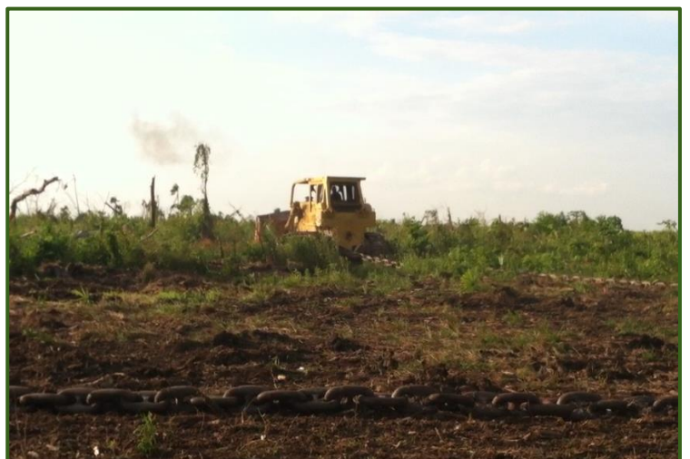
First Heavy Bulldozer heads off into light bush to begin clearing
