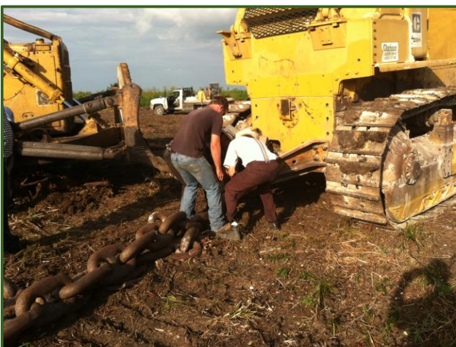
Chain being attached to Heavy Caterpillar D-9 Bulldozer
